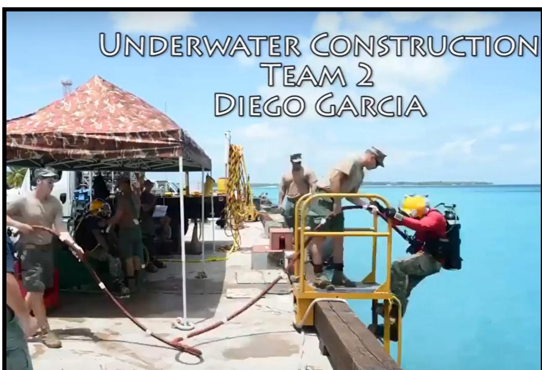
UTC construction site in Diego Garcia
